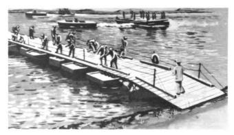
Figure 6-49. Ponton bridges. Light and heavy-weight ponton bridges are employed by the Soviet Ground Forces. The LPP light ponton bridge (above) can carry up to 40 tons, and the heavy TPP (below) carries up to 70 tons. Each ponton is carried on a single truck.
